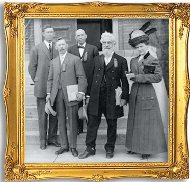
In 1869, Norman J. Colman, second from right, suggested a School of Journalism.
